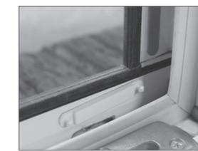
4. Place the magnet holders (2) with the magnets on the small metal plates fixed in the window frame.
