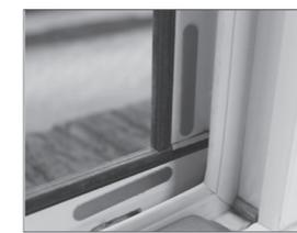
3. Attach the small metal plates (3) inside the window frame: To do this, stick 2 small metal plates in each of the corners of the frame.
